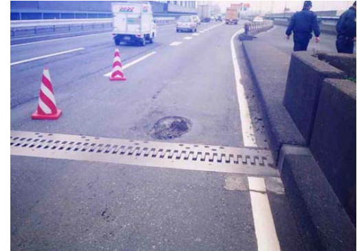
Damage of Pavement on the Crack
