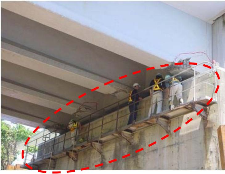
Example of providing the walkway
