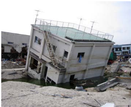
Fig. 12 Tilting by scouring
