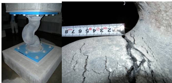
Fig. 8 Lead damper cracked
