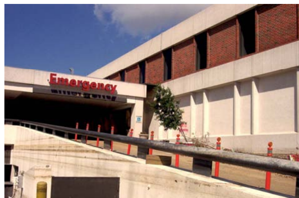
MCEER research is strengthening critical infrastructure. Photo courtesy of MCEER.
