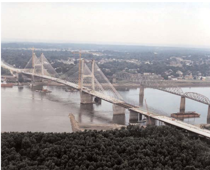
Emerson bridge nears completion in 2003 (bridge in the background has since been demolished). Photo courtesy of MoDOT, http://www.modot.org/southeast/projects/bridge/index.htm#gallery .
