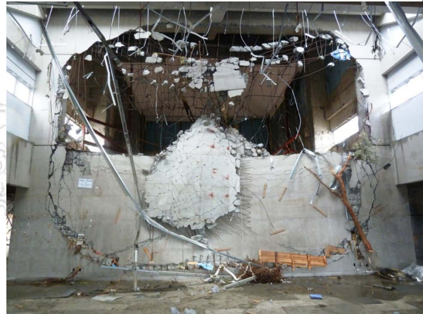
Rikuzentakata Takada Matsubara Building Shear Wall Blowout
