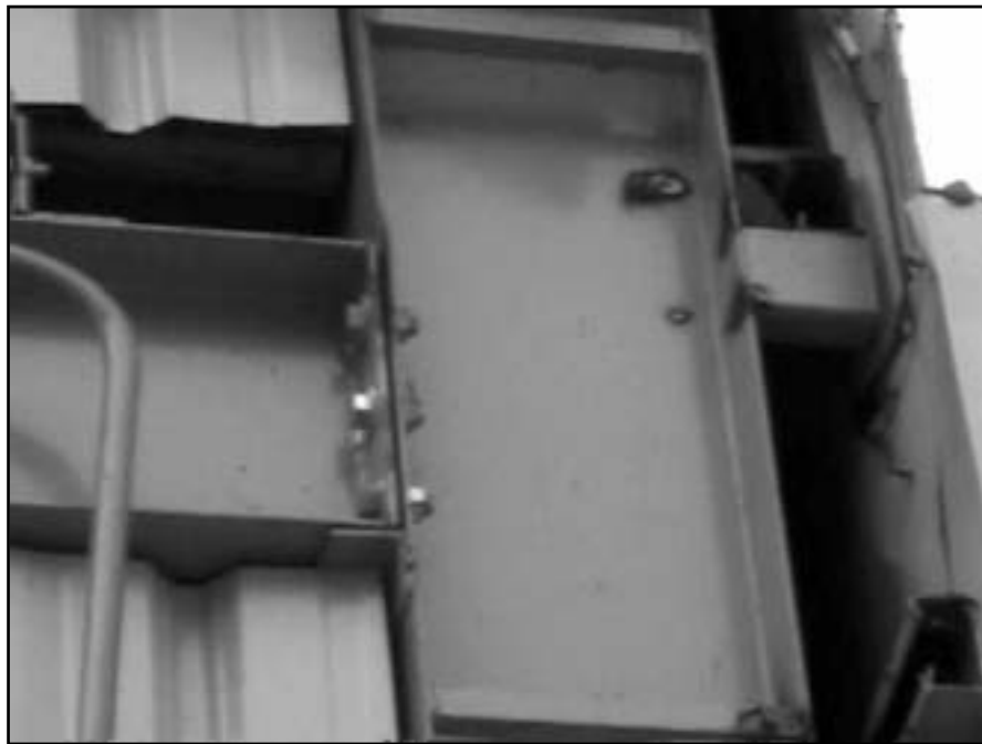
Figure D-4 Bolted End Plate Connection in Light Steel Frame Building Showing Evidence of Local Yielding
