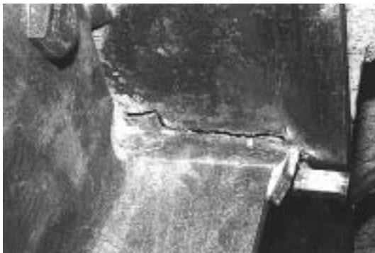
a. Fracture at Fused Zone
