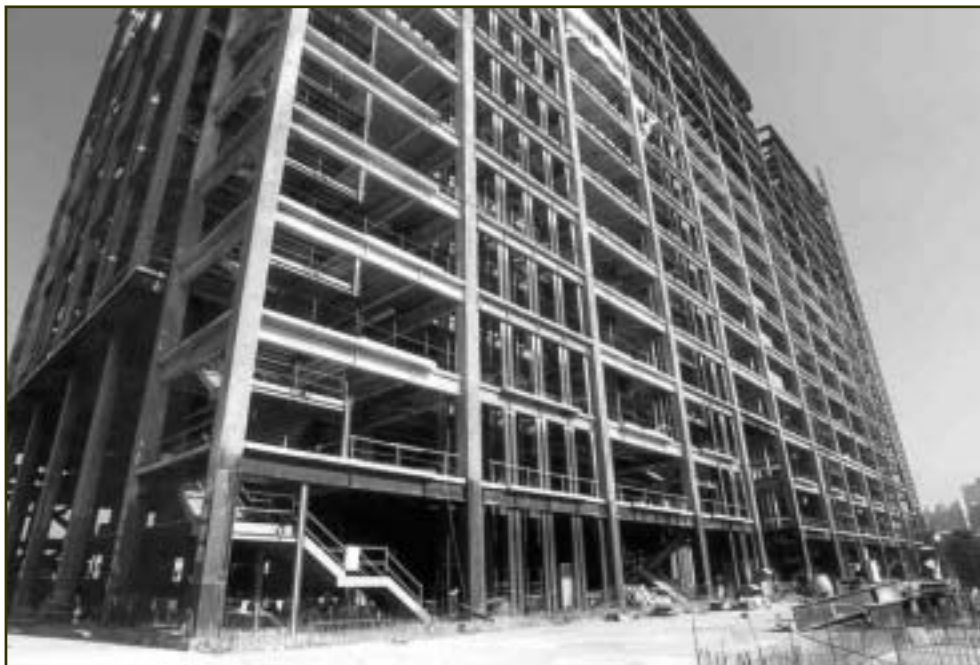
Figure D-2 Typical Taiwanese High-Rise Structure under Construction in Tiachung
