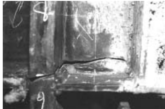
a. Fracture Progresses into Column Web
