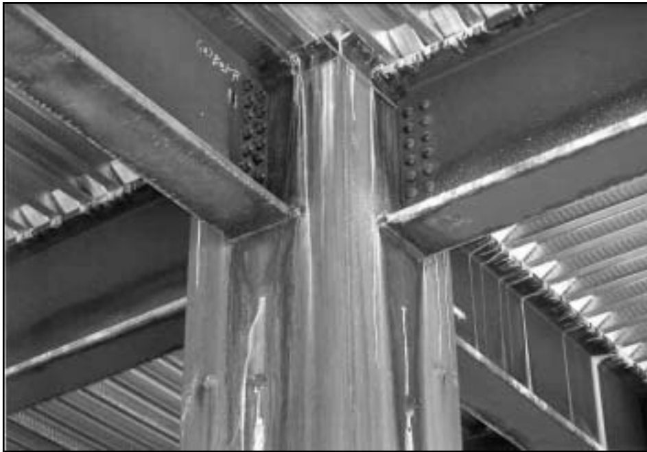
Figure D-3 Welded Connection Detail of Beams to Box Column
