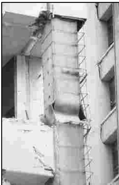
Figure 5-2 Damage to Steel Frame Column, Mexico City Earthquake, 1985
