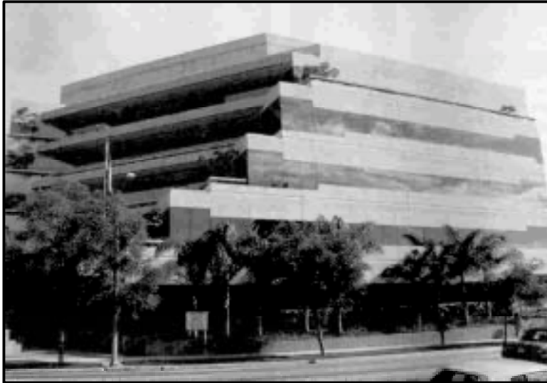
Figure 2-6 WSMF Building with Setbacks
