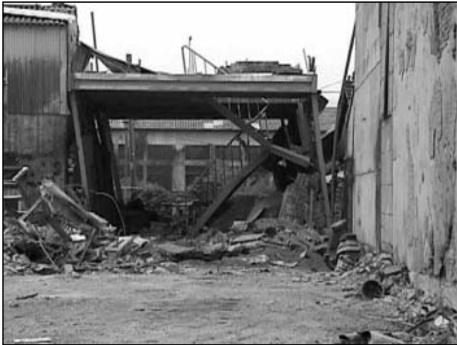
Figure D-1 Permanent Lateral Displacement in Small Steel Frame
