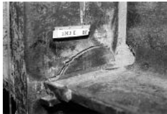
b. Column Flange "Divot" Fracture
