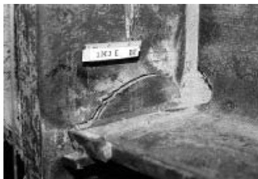
b. Column Flange "Divot" Fracture
