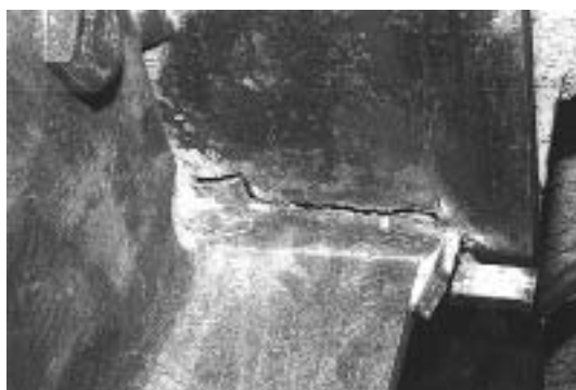
a. Fracture at Fused Zone
