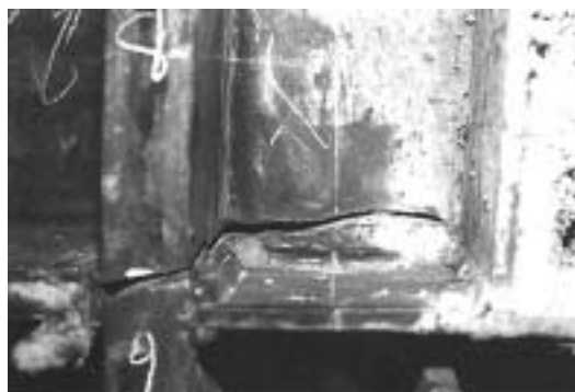
b. Fracture Progresses into Column Web
