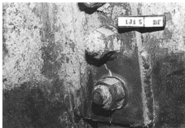
Figure 1-5 Vertical Fracture through Beam Shear Plate Connection
