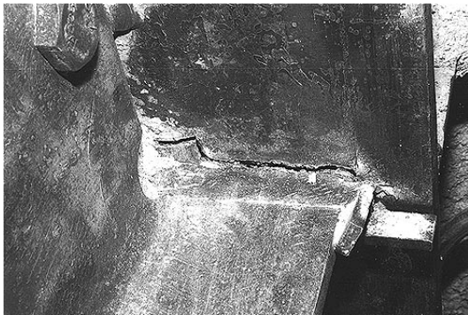
a. Fracture at Fused Zone
