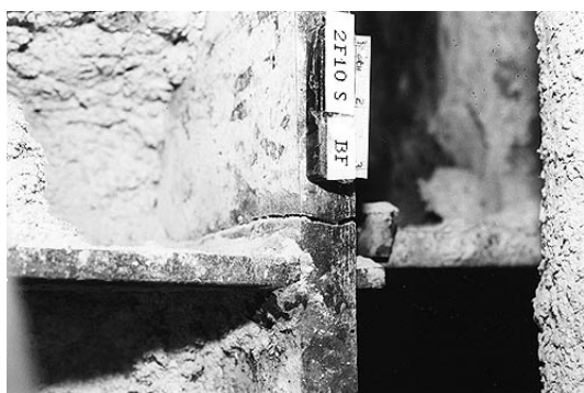
a. Fractures through Column Flange
