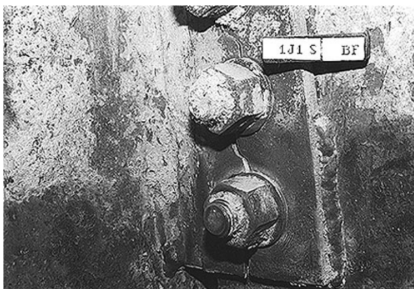
Figure 1-5 Vertical Fracture through Beam Shear Plate Connection
