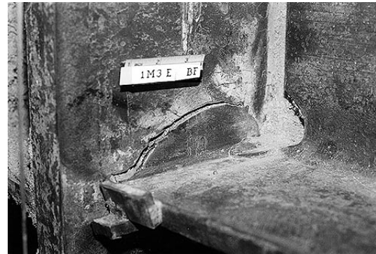
b. Column Flange "Divot" Fracture
