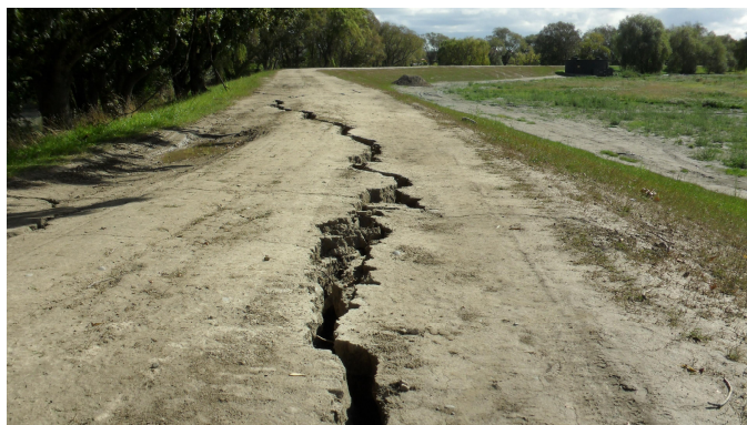
A lateral spread crack running along the crest of a levee in Kaiapoi, just north of Christchurch. Courtesy of R. Green, Virginia Tech.
