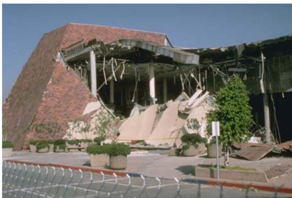
Department store that partially collapsed in California's 1994 Northridge earthquake; punching shear failure was observed. Source: J. Dewey, U.S. Geological Survey.
