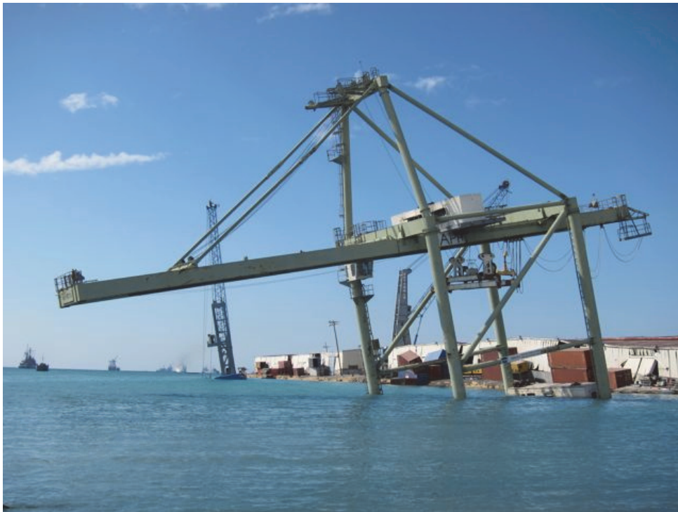
Figure 2-4 Submerged 15-meter gauge A-frame container crane (foreground) and mobile crane (left center, background), Port de Port-au-Prince, following the 2010 Haiti earthquake. A second, apparently undamaged, mobile crane is shown upright (right center, background).
