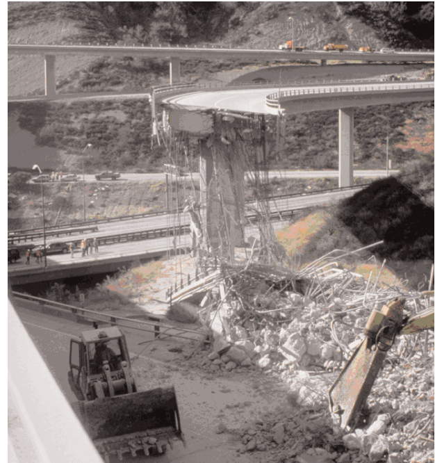
Freeway bridge collapse, Northridge earthquake, 1994. Credit: Mehmet Celebi, USGS
