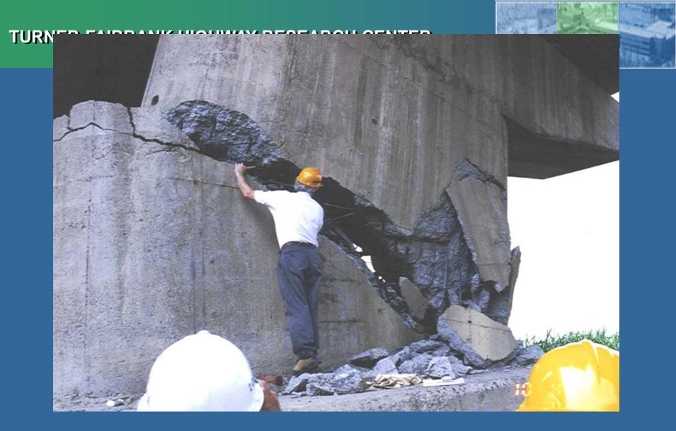
Shear failure in pier of Wu-shi bridge, Chi-chi Earthquake, Taiwan, September 1999
