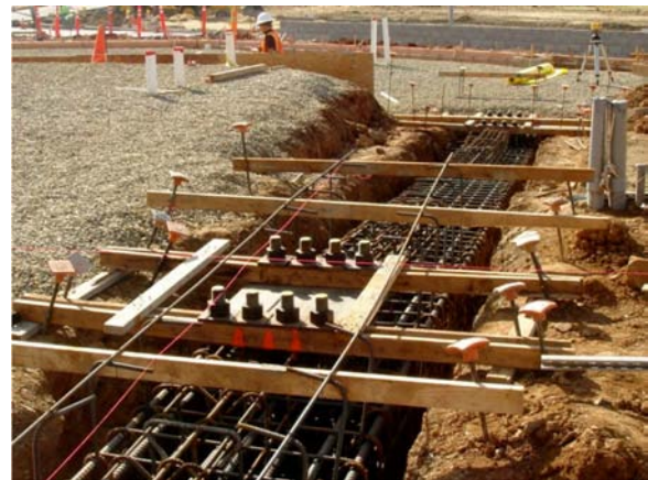
Figure 6-1 - Concrete grade beam connecting adjacent column steel special moment frame bases.
