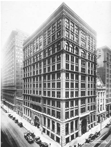
Figure 2-1 - The Home Insurance Building – Chicago, IL, 1885, an early skyscraper.
